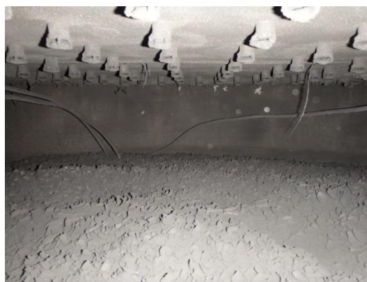
Fig. 12. Graded bed fouling.
